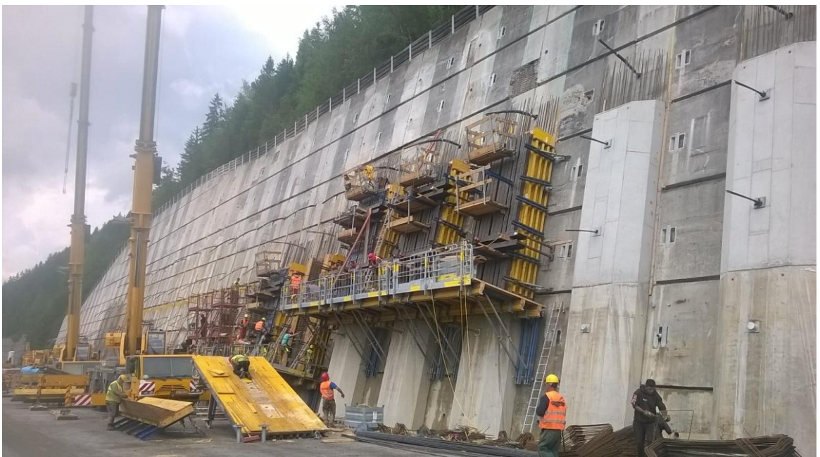
A10-Tauernautobahn, RFB Salzburg, Ankerwand Egger
